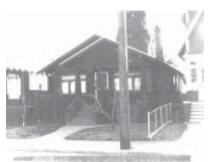
Approved by the Planning Department in 1993. Second story added, front porch partly enclosed and entire building covered with vinyl siding. Original surfaces were wood shingles. Horizontal aluminum slider windows added which are inconsistent with the original Craftsman style
