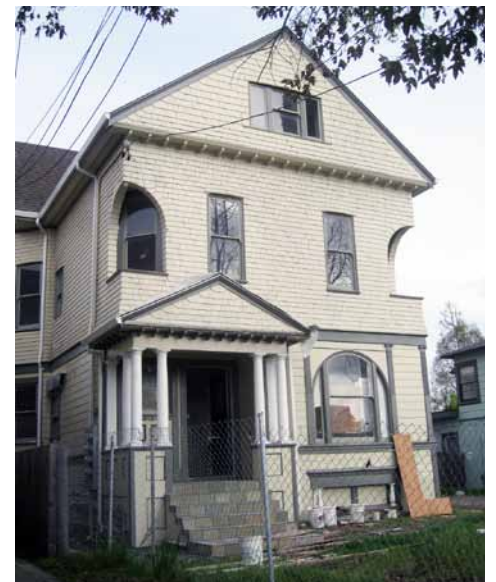
2010 photo showing renovation nearing completion. Note replication of original details: slight bulge of gable above window, upswept shingle courses at gable edge, and sawtooth shingles on bottom course. (Photo: Betsy Mathieson.)
