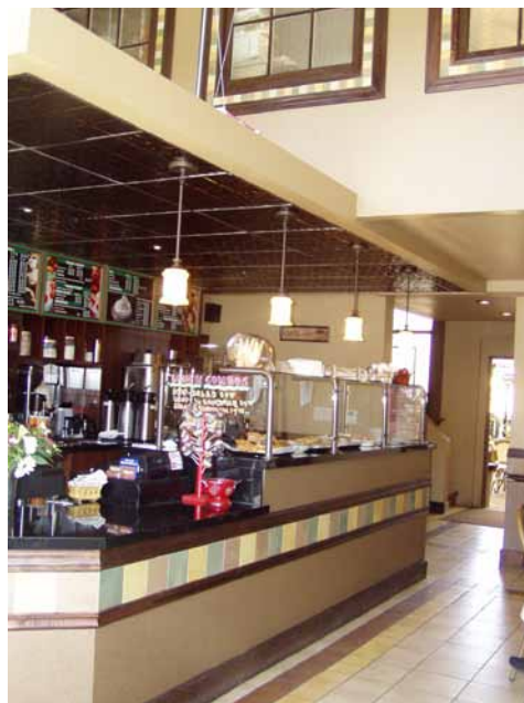
Traditional tilework on the floor and dark wood trim work is reminiscent of the building’s 1916 vintage. Stamped sheet metal ceilings and period light fixtures complete the period ambience. (Photo: Jerri Holan.)
