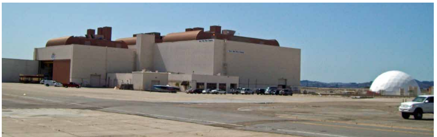
Encompassing 63,000 square feet, Building 024 and its smaller satellite Building 024A cost $19,251,343.00 to construct. Inside, there are three large high-bay aircraft painting hangars, each one about 130-ft square. (Photo: Dave Duffin.)
