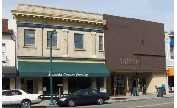
The east end of the City Market Building was sullied by stucco in 1954, rendered smooth and deprived of detail. (Photo: Judith Lynch.)
