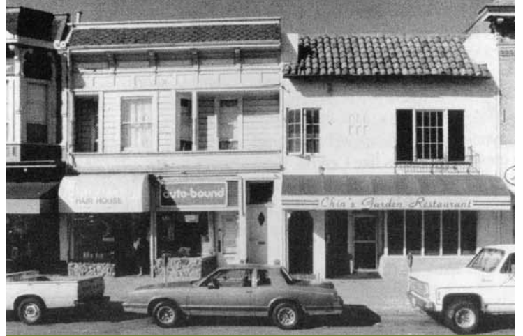
The Hally Buildings 2313 and 2315 Santa Clara Avenue built in 1894 and 1892 by George MacRae originally had mirror image façades. 2315 was altered with stucco and a tile roof in 1934.
