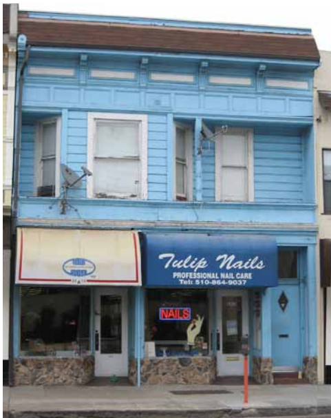
Peeling paint, stone siding, and mismatched doors and awnings from bygone tenants graced the old storefront.
