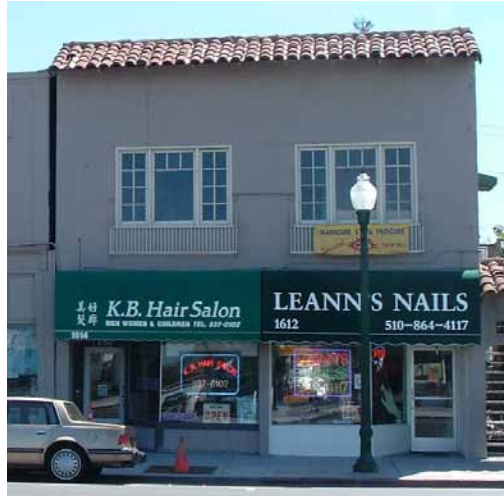
Plywood and other 'alien' materials were removed from the tiled bulkheads, which were reconstructed. The transoms had been poorly maintained; some of the windows were painted over, and others were smothered with plywood.
