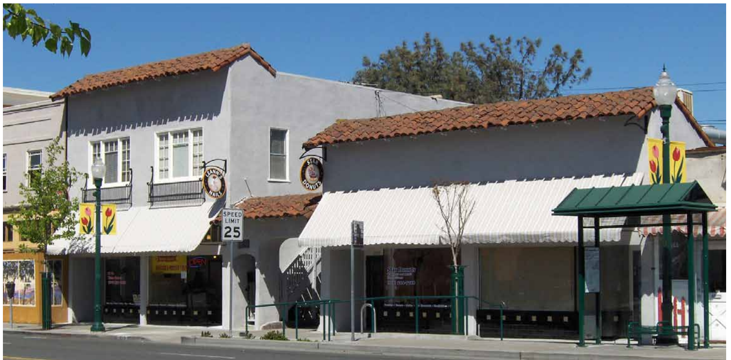
The award-winning rejuvenation of the Gohnauer Building-West End Market, 1610-14 Webster Street, and its neighbor, of 1606-08 Webster Street. Owner Charlie Ma went ahead with the upgrade project because “I wanted to make the city look better and to get more business for the store owners who are my tenants.”
