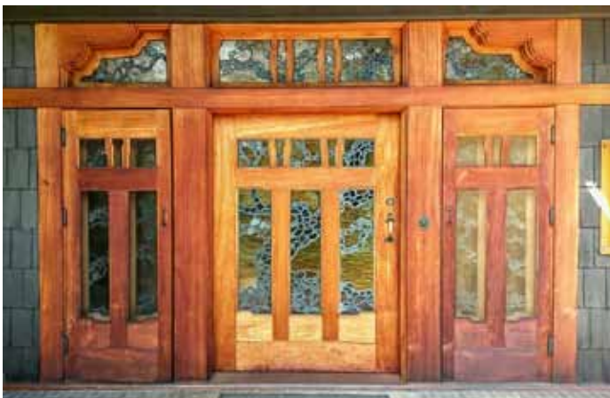
Front entry door, operable sidelights and fixed transom windows are filled with a stained glass masterpiece. Image: Wikipedia.com.
