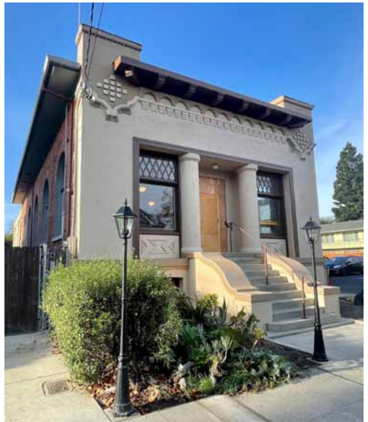
Facade remodel as of November 1st. Waiting on the entrance door, which will be a solid oak door with a beveled oval glass from 1900 that has matching dentils as the windows. Running down the side, the fascia will be exposed and 18 corbels installed to match the front.
