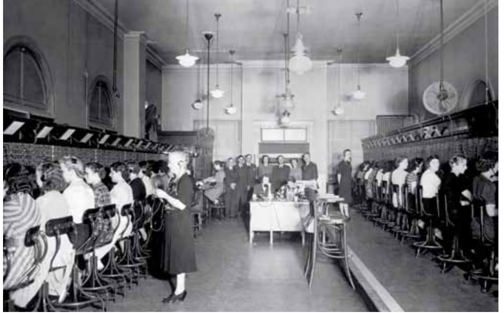
The Sunset Telephone and Telegraph Company's switchboard circa 1930s.
