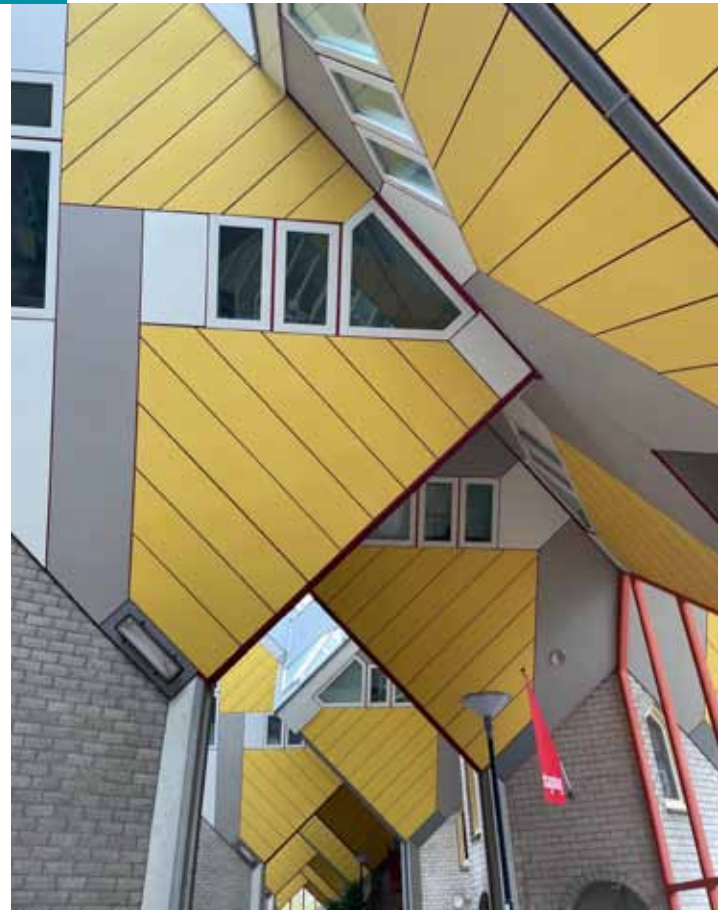
▲ The complex, also known by its nickname "Blaak Forest", is a modern architectural icon that cannot be missed when visiting Rotterdam.
