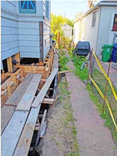
Outside photo of forms for the new foundation.
