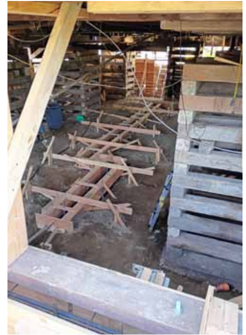
New foundation, temporary supports, and forms for new footings.
