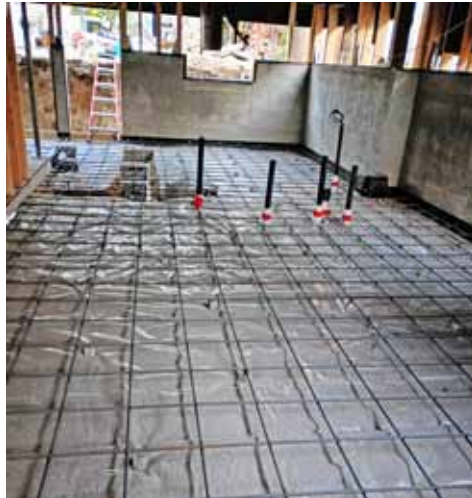
Basement with rough plumbing and rebar for basement slab.
