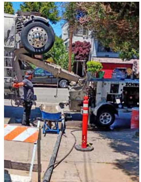
Concrete being poured for foundation.
