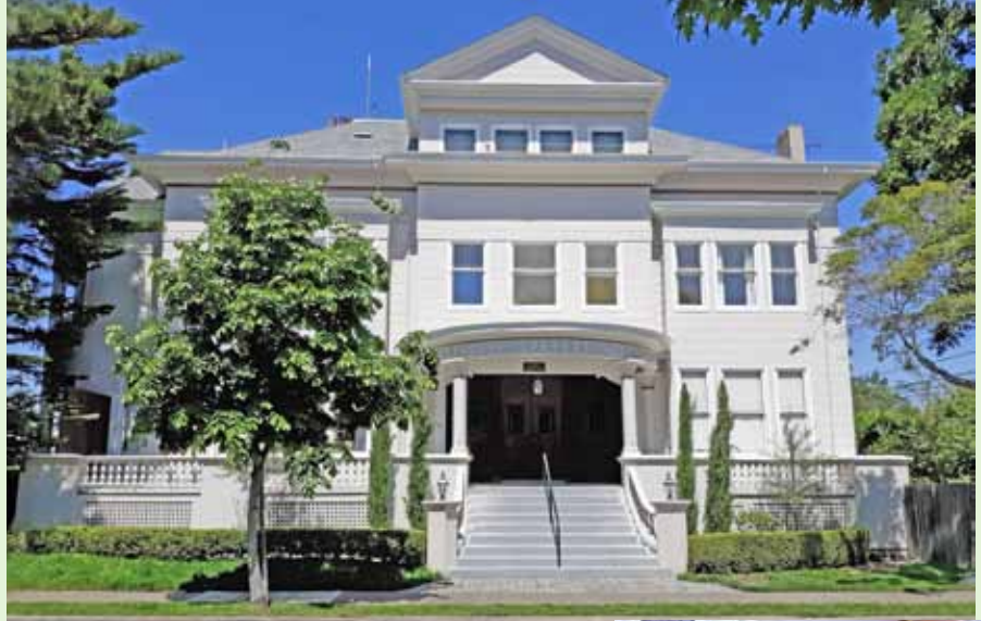
After updates and repairs, the home received a fresh coat of paint giving the home a renewed presence on the street.
