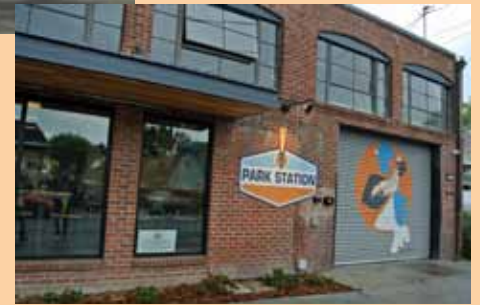
Today the south wall roller door features a mural, the company logo, and an updated color scheme.
