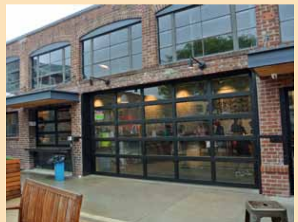
Two original metal roll-up doors were replaced with glass roll-up doors to maintain an inside/outside connection.
