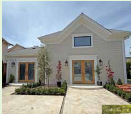
The original carriage house was rebuilt and modified to serve as an ADU.
