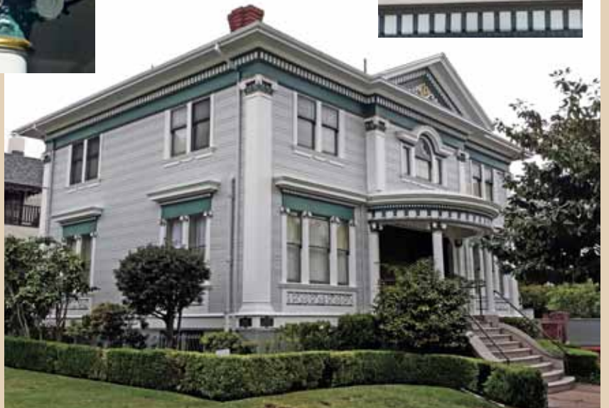
Facade after painting at west corner of Paru Street and Dayton Avenue.
