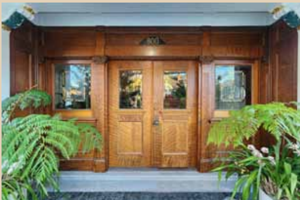
Refinished front door.
