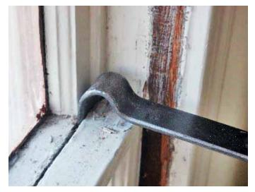
If the window is stuck in the frame, it is probably held by an exterior paint seam that you can't reach. To break this seam insert your pry bar between the upper and lower sash sides, as shown and pry gently. There will be a little "pop" when the outside seam breaks. With both side seams broken, the window should release.
