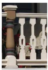
Right: Detail of the porch. Metal railings and columns were removed and replaced with generous Newell posts and carved pickets.
