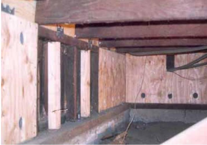
Cripple wall retrofit, including plywood sheathing and load path connectors (Credit FEMA G225).
