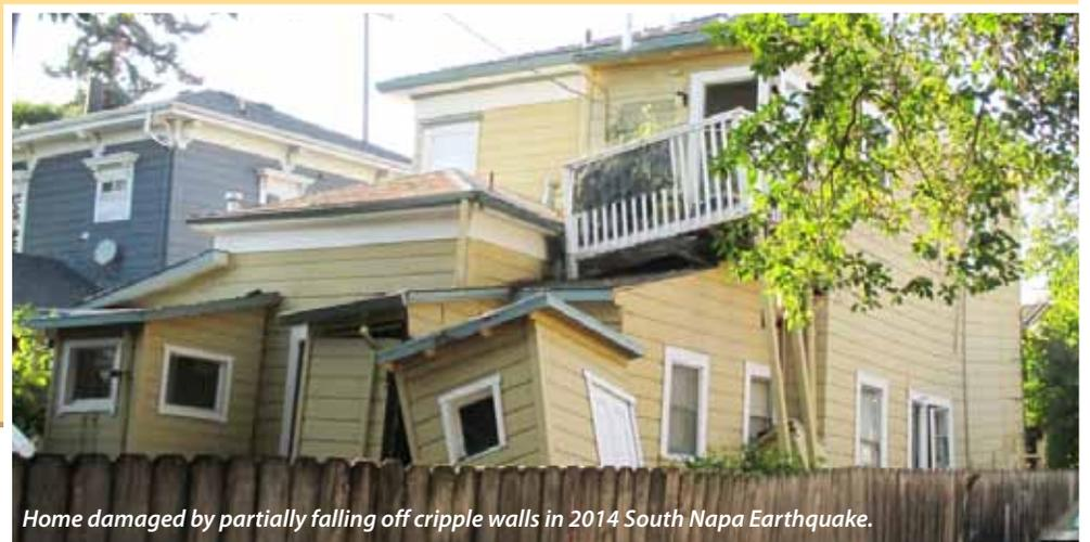
*Home damaged by partially falling off cripple walls in 2014 South Napa Earthquake.*
