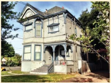
Left: This Lafayette Street residence has been refreshed with extensive restoration from the foundation up. Wood trims, original windows, the front door, were retained. When that option was unavailable a complete replacement like for like was implemented.
