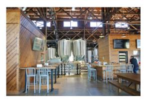
Left: Inside large wood trusses, posts and beams are all exposed, a new concrete floor in a portion of the building was installed and the two tenants have sensitively adapted their businesses to the old structure (Almanac Brewery shown in photo).
