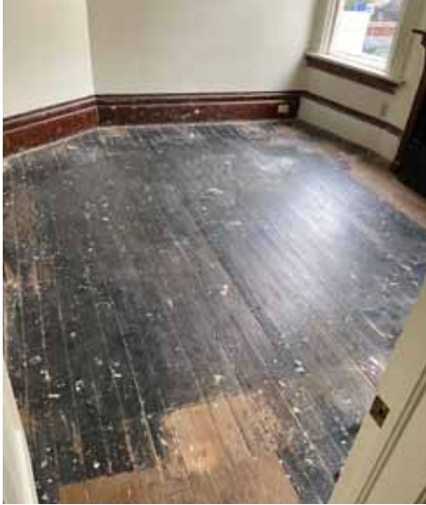
Parlor floor before restoration. Brenden removed 100 years of paint and old flooring, and now the original fir floors are exposed in both the parlor and the bedroom.
