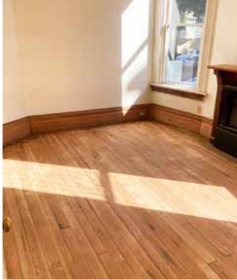
Parlor floor before restoration. Brenden removed 100 years of paint and old flooring, and now the original fir floors are exposed in both the parlor and the bedroom.
