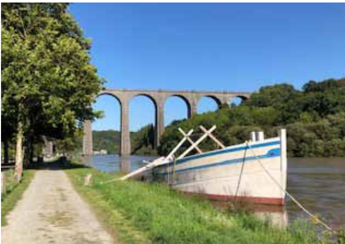
▲ 1866 stone viaduct, its twelve arches connect the valleys on either side.
