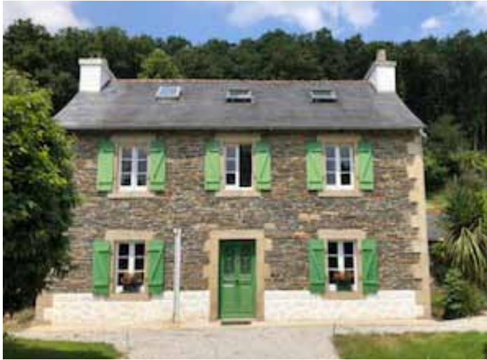
▲ The granite and slate house in Brittany, Finistère.
