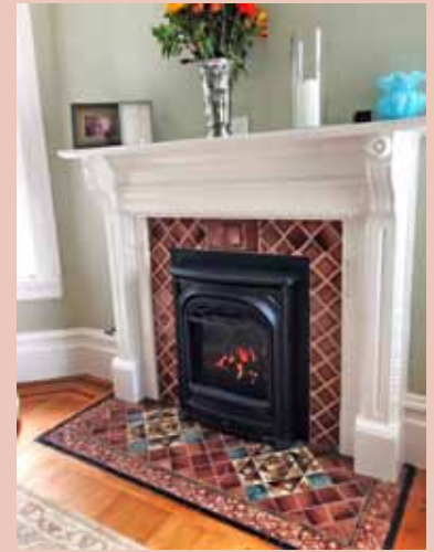
Above: The original fireplace was kept intact and was outfitted with a new gas insert. Damaged tiles were replaced with original tiles from a matching fireplace onsite.
