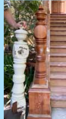
Detail: Surviving newel post was the design clue and set the stage for the complete design of the staircase restoration.
