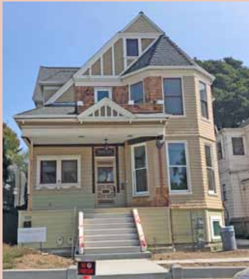
Above: The front bay windows needed refurbishing and the front porch was partially covered with cement. Some shingles needed to be replaced due to water damage.
