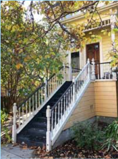
Left: The staircase before the demolition had rotted and broken "off the shelf" posts and balusters installed in the 1980s when the concrete foundation was put in.
