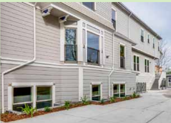
Left: Rear addition with new basement light wells.
