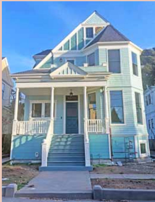
Below: The front porch was resurfaced and maintained the historically accurate 30-inch railing height. The newel posts were custom made to match the interior stairs.
