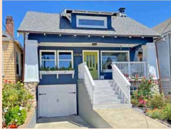
The house is transformed by incorporating Craftsman details the beaded porch ceiling, wood cladding and river rock stone veneer on the front columns and custom made garage doors, among many other upgrades.
