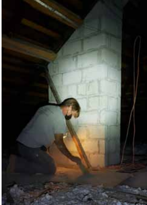
Replacement of attic chimney. Image: Jason Wady.
