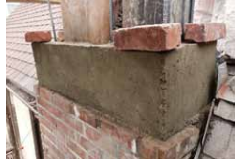
Concrete installed around rebar and straps. Image: Jason Wady.
