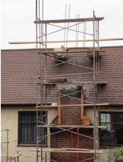
Damaged section removed and rebar added. Image: Jason Wady.
