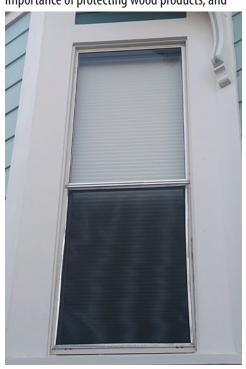
Aluminum windows were very popular and used extensively as an inexpensive waterproof solution when replacing rotted wood windows in older houses.
