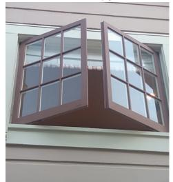
This new wood casement window replaced a rotted double-hung window. The style still matches the original house design but offers a more functional use of the same opening.
