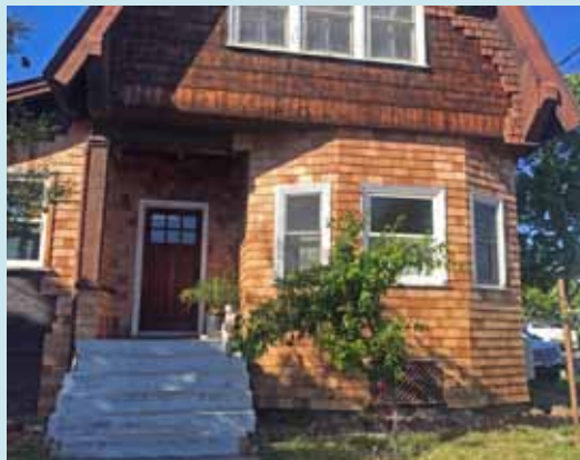
The bottom shingles have been replaced with new cedar shingles.
