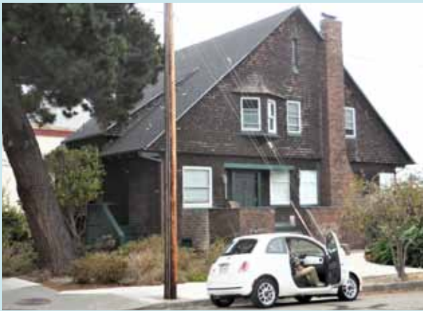
2000 Clinton prior to exterior restoration.
