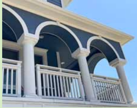
The open porches on these town-homes feature curved openings, corbels, wide trim work and variety of column styles reminiscent of the Victorian era.
