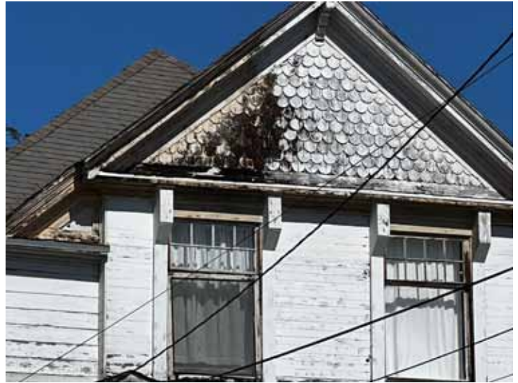
Here's an example of dry rot causing structural damage underneath. Image: Devon Westerholm.
