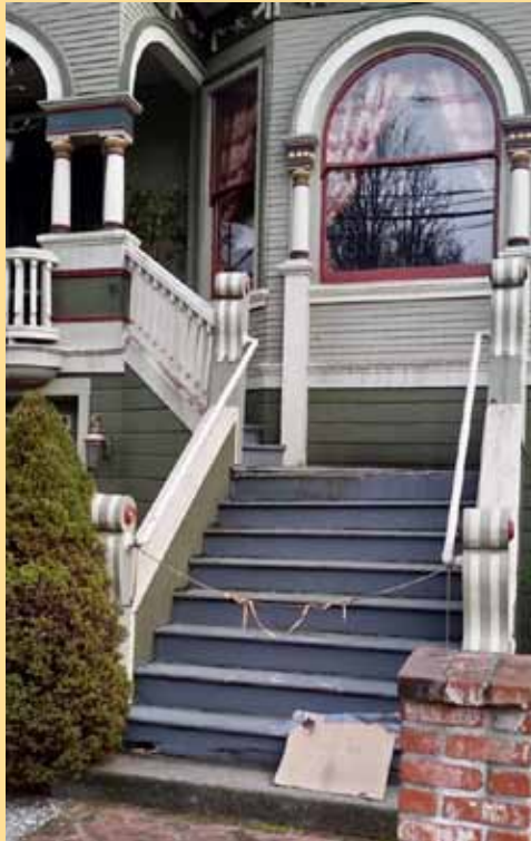
The front staircase was rotted and completely worn so it had to be ripped out and replaced.
