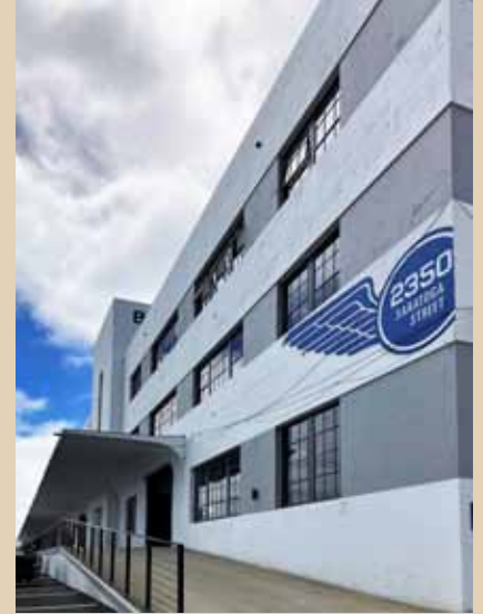
The original design of the building was preserved: from the modern overhang above the loading dock and the roll up doors, to the industrial steel sash windows that were reglazed.
