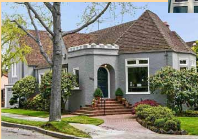
The 1928 split-level house before the renovation. Top-of-mind for the homeowners were respect for architectural integrity, consistency of design and quality of materials.
