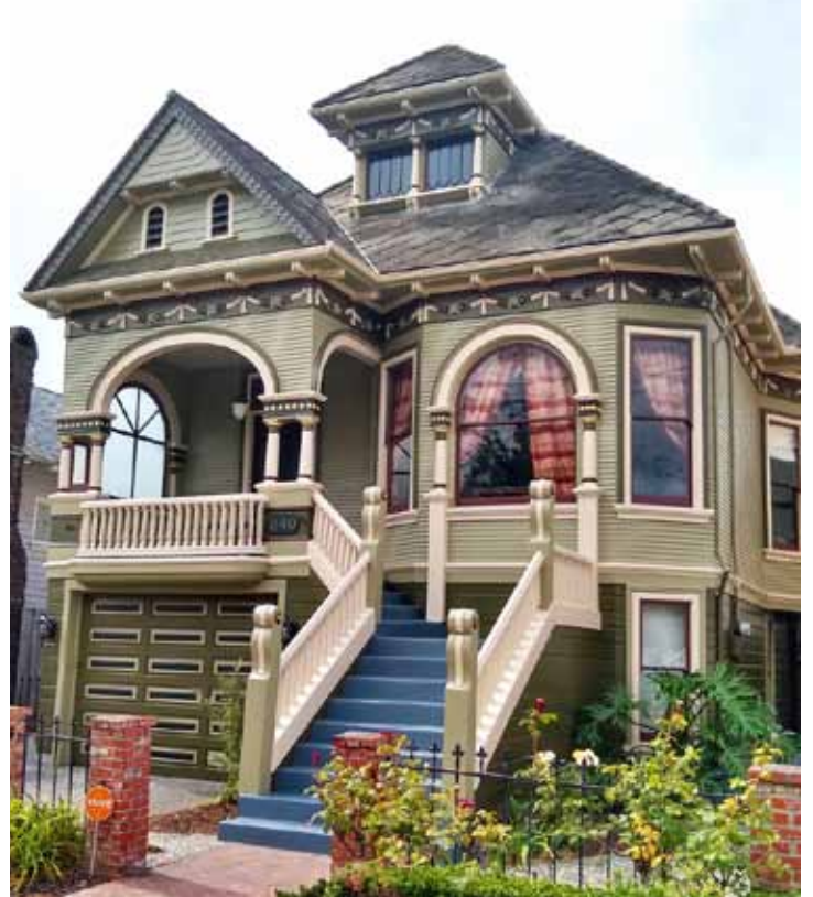
This Marcuse & Rimmel Colonial Revival shows off its gorgeous architectural details, some of it newly restored with a seven color paint scheme and an abundance of gold leaf.
