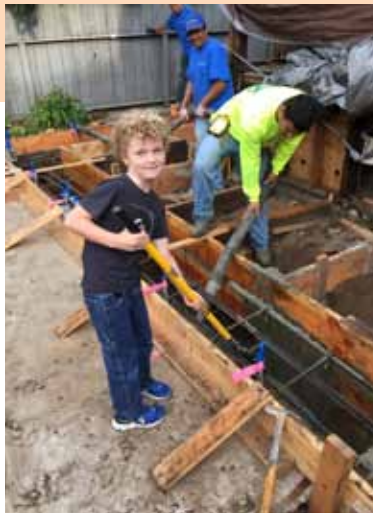
The owners' son helped with the foundation work.
