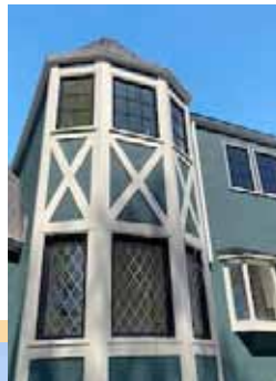
Left: The primary bathroom addition on top of the octagonal breakfast nook is bound by exterior half-timbering.
