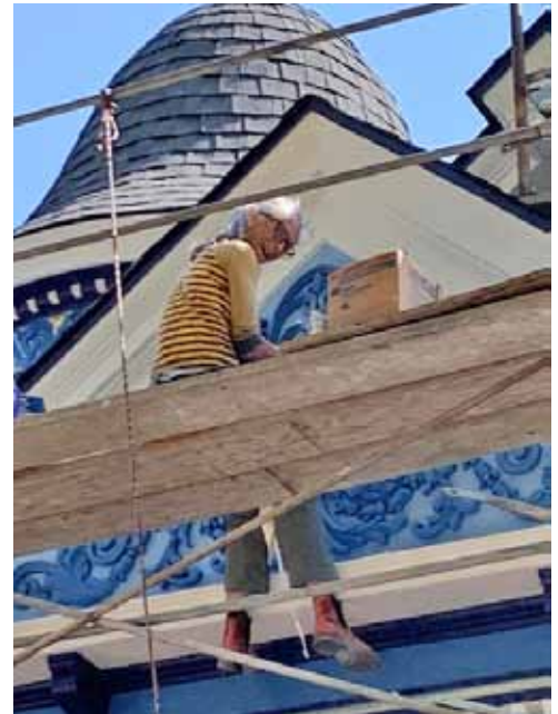
Lorna at work on the facade of the house.
