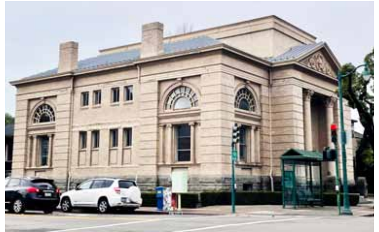
The 1903 Carnegie Free Library Building, at the corner of Santa Clara Avenue and Oak Street, has been closed and vacant for over 20 years. The Strategic Plan calls for identifying reuse opportunities for the former Carnegie Library.
