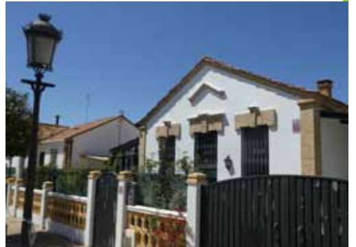
▲ On this one story house, its unique brick lintels feature long keystones.
