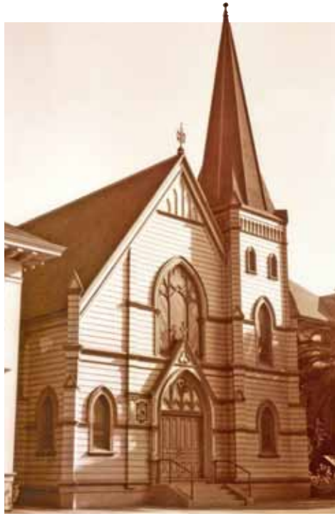
A historic view of the Lafayette Street elevation in 1938. Image: Immanuel Lutheran Church.
