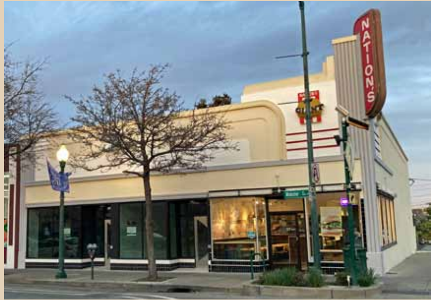
The restored storefronts and molding relief are once again seamlessly integrated into the original structure.
