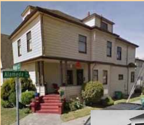
The house retained its original style but was completely covered in aluminum siding, losing the original exterior window and door frames in the process.
