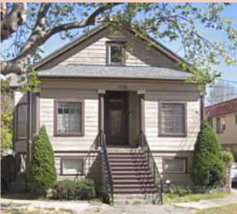
The front porch was enclosed to enlarge the two upstairs units and accommodate their kitchens on either side of the front door.
