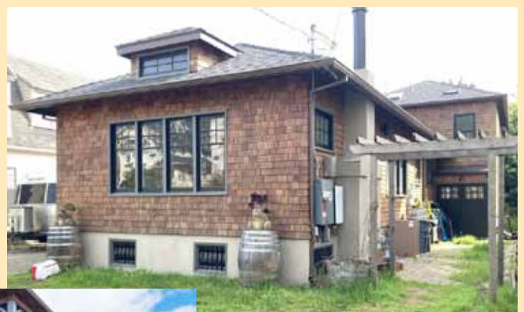
New, architecturally appropriate windows, new cedar shingle siding, and a brand-new roof allowed the addition to tie in seamlessly with the original craftsman aesthetic.
