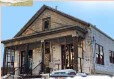
Restoring the original porch was a huge undertaking. In the process, the original colored paned transom window was uncovered and restored.
