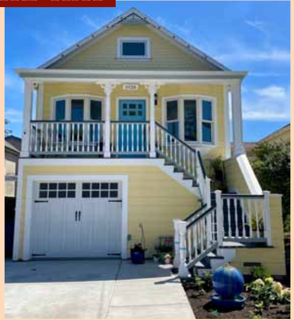
New siding, custom woodwork and trim throughout the front porch provided the Victorian finishing touches.
