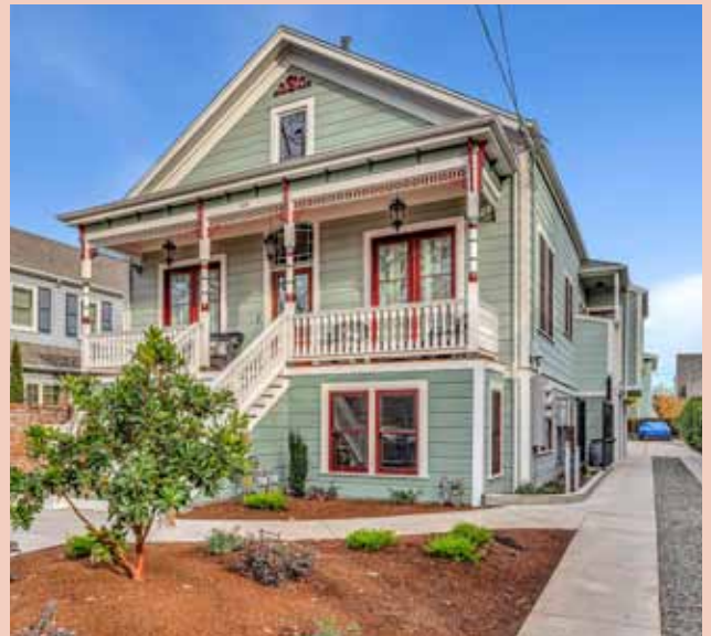
The newly restored house stands out with its showpiece porch finished in tongue and groove Douglas fir and custom millwork.
