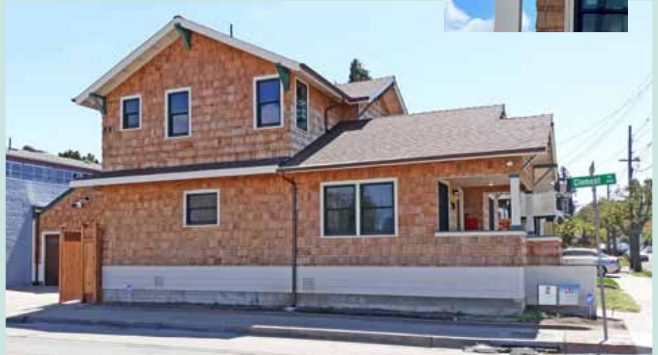
New cedar shingles in a ribbon course design were added throughout the exterior walls, and knee brackets were incorporated to the front and side gables.
