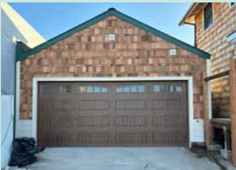
The garage was completely rebuilt to fit two cars and add much needed storage. The wood shingles, flat front and gable design is all in keeping with the house's original style.
