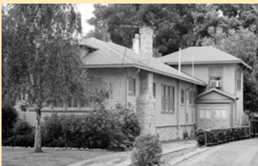
The Craftsman front remains untouched. Here the small garage would've fit a Model T. Image: Alameda 1979 Survey.
