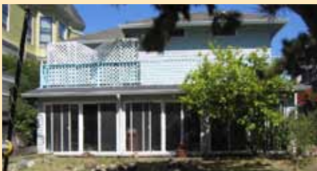
The 1980s remodel enclosed the back deck with aluminum floor to ceiling windows and the shingles were painted an unappealing light blue color.
