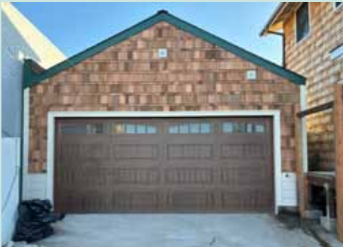
The garage was completely rebuilt to fit two cars and add much needed storage. The wood shingles, flat front and gable design is all in keeping with the house's original style.
