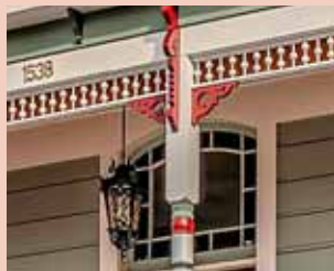
Restoring the original porch was a huge undertaking. In the process, the original colored paned transom window was uncovered and restored.
