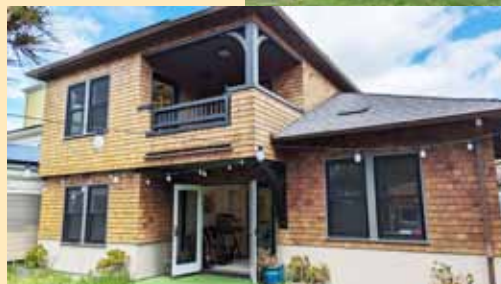
New, architecturally appropriate windows, new cedar shingle siding, and a brand-new roof allowed the addition to tie in seamlessly with the original craftsman aesthetic.
