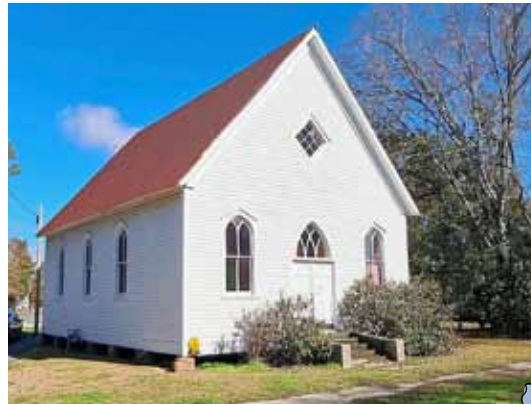
The colored glass windows of the 1904 converted church create a colorful light display inside the one room rental. Image: David Bock.
