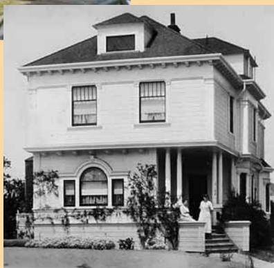
Circa 1910. The large Palladian window and rounded columns on the entry porch are reminiscent of the Colonial Revival style popular at the end of the 19th century. Image: Alameda Museum
