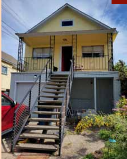
The house was raised and stuccoed, aluminum windows installed and cement stairs and wrought iron were added to "modernize" its appearance.
