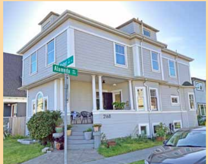
Fortunately the original windows were not modified but needed to be replaced, so they were recreated to match the original double hung style with top leaded panes, and the curved glass in the bay.
